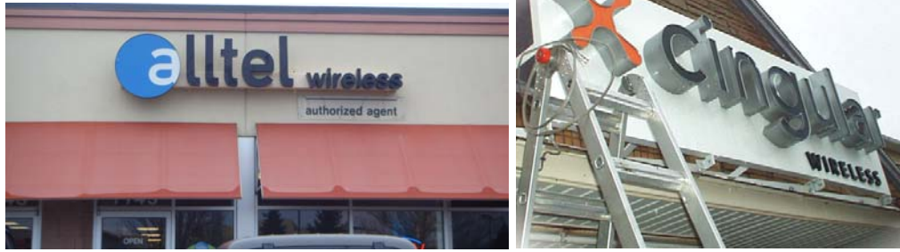
Figure 1: These examples of Channel Letter Signs are raceway mounted and pin-mounted, respectively.
